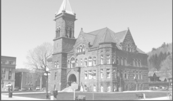
Barbour County Courthouse Renovations
