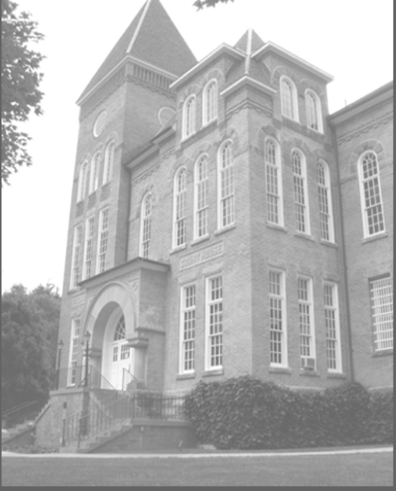
Pocahontas County Courthouse Renovations
