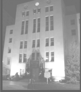
Harrison County Courthouse Renovations
